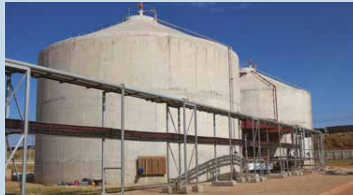
NEW 50 ML/DAY MODULE 2 AT WELGEDACHT WATER CARE WORKS
